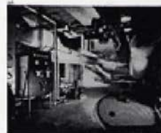
Secretariat has four pipe galleries plus added equipment in basement, each supplying floors as shown at right. Buildingwide tons of levers at each mechanical floor are used for fresh and exhaust air. Photo above shows part of a mechanical floor, which permits concentration of most heating, air conditioning, electrical, telephone and other such equipment.
