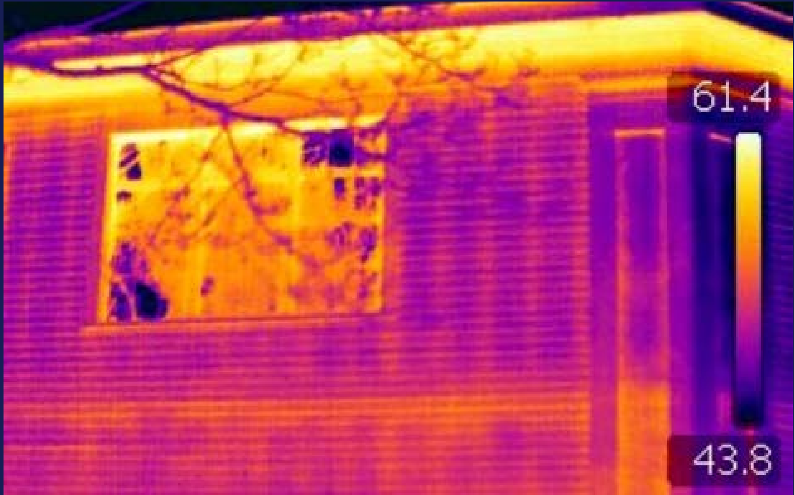
Image 9: Infrared image highlighting the thermal bridging caused by the metal studs
