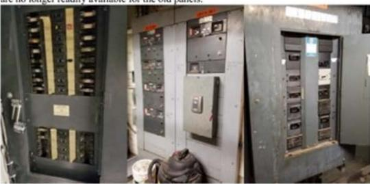
In older portions of the building, the existing electrical closet doors are small, and generally cramped. There are some working clearance issues, some of which are rather severe. There are a number of electrical panels located in corridor walls. This is not allowed by current guidelines. When renovating, these panels will have to be moved out of the corridors. In general the existing panels and electric closets will not support renovation.
