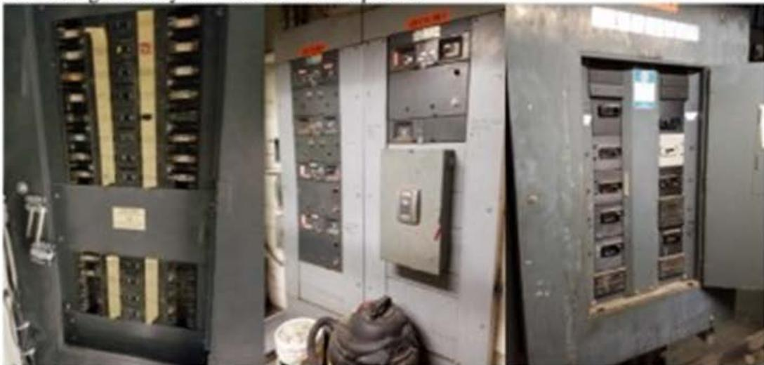
In older portions of the building, the existing electrical closet doors are small, and generally cramped. There are some working clearance issues, some of which are rather severe. There are a number of electrical panels located in corridor walls. This is not allowed by current guidelines. When renovating, these panels will have to be moved out of the corridors. In general the existing panels and electric closets will not support renovation.
