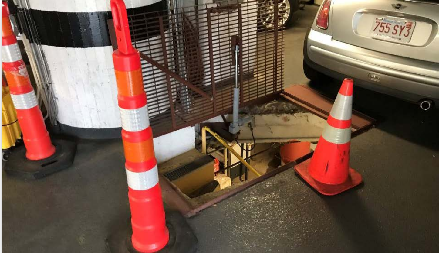
Lower Level Basement Access Open Grated for Boiler Ventilation
