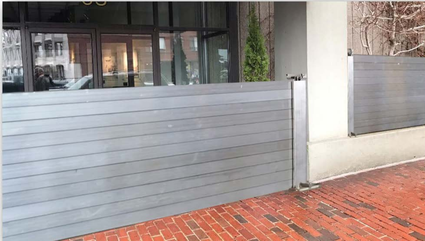
Flood Barrier at Entrance, Garage and Basement Access
